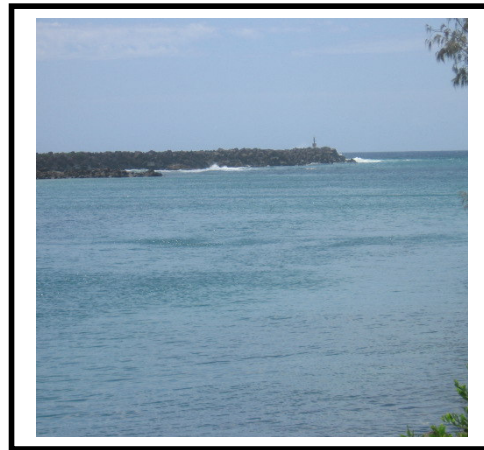
The Brunswick River with wall that extended the bar out beyond the beach.
