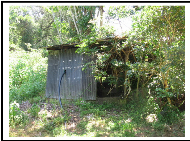
The Engine Room on the creek for pumping water up to the top tank. It housed a big diesel engine and a belt driven piston pump that drew water from the lower pool in the creek.
