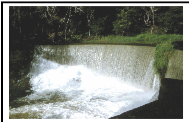
Wilsons Creek Weir in Floodtime
