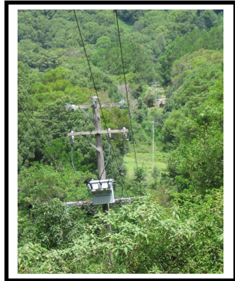
Electric Power Line Cutting Across the Creek from Browns Place
