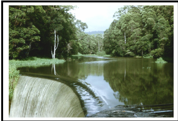
Wilsons Creek Weir holds back several kilometres of water
