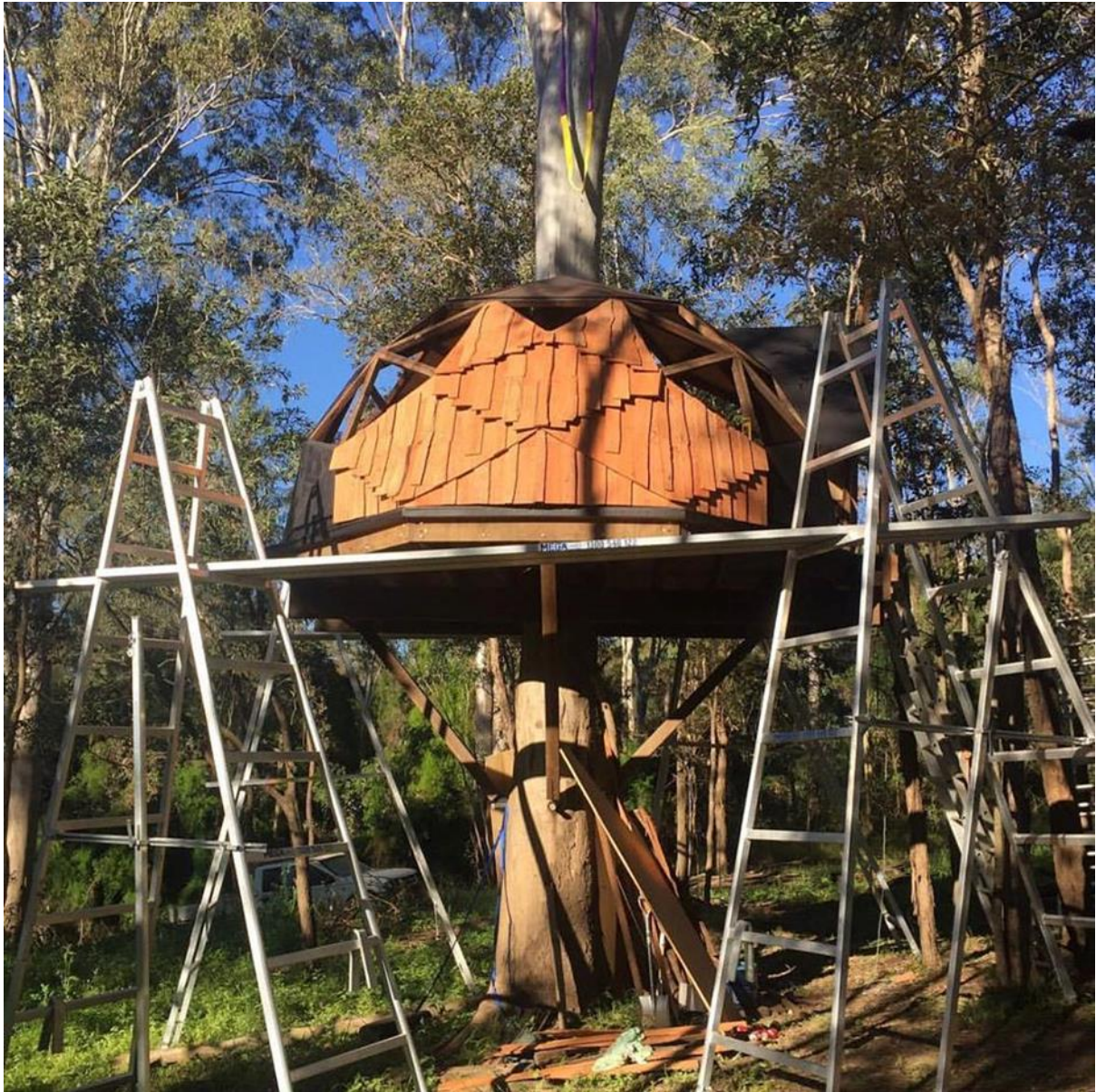
Shingles going on the Geodesic Dome
