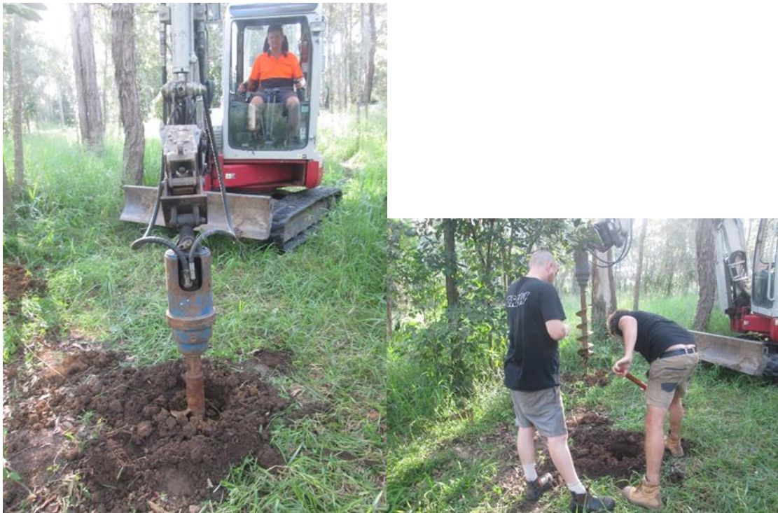
Anthony and Pat digging out the twelve holes for the steel stirrups to be concreted in for the twelve vertical posts which will support the deck. The deck is twelve sided.
