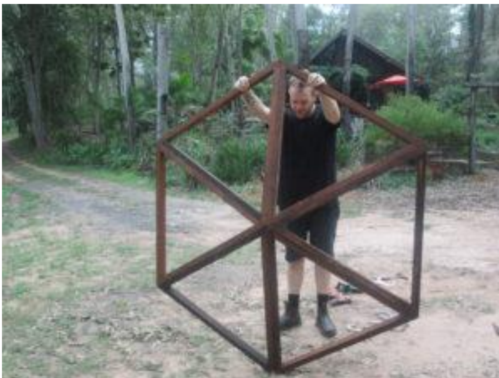
Triangles of wood were screwed together for a portion of the roof the Geodesic Dome
