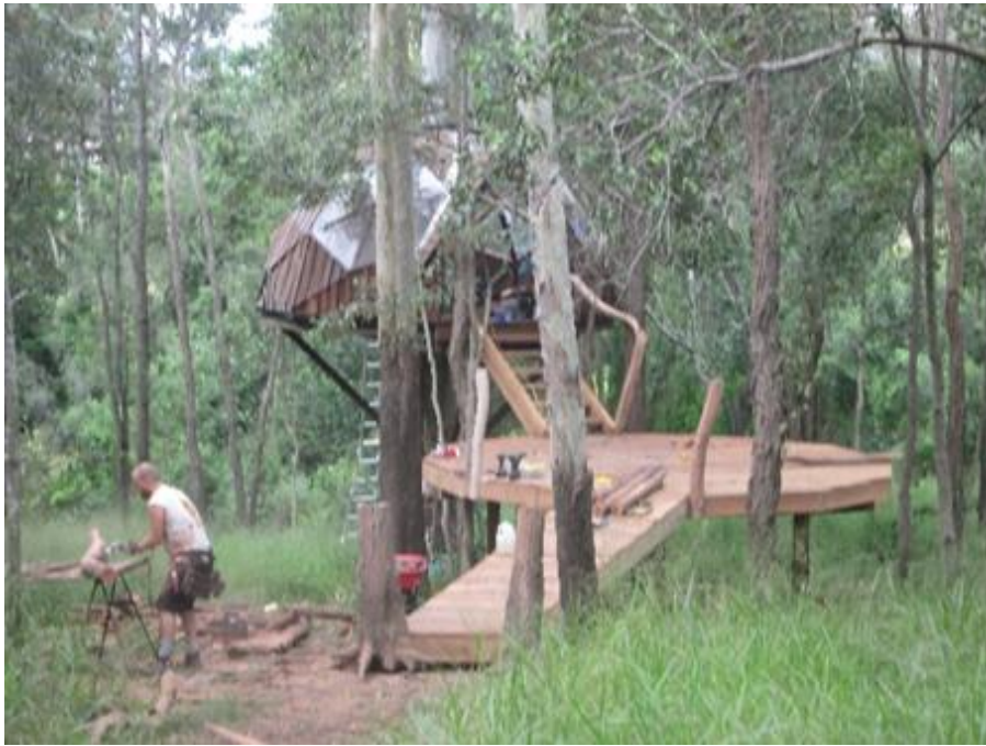
The deck as it is in April 2018
