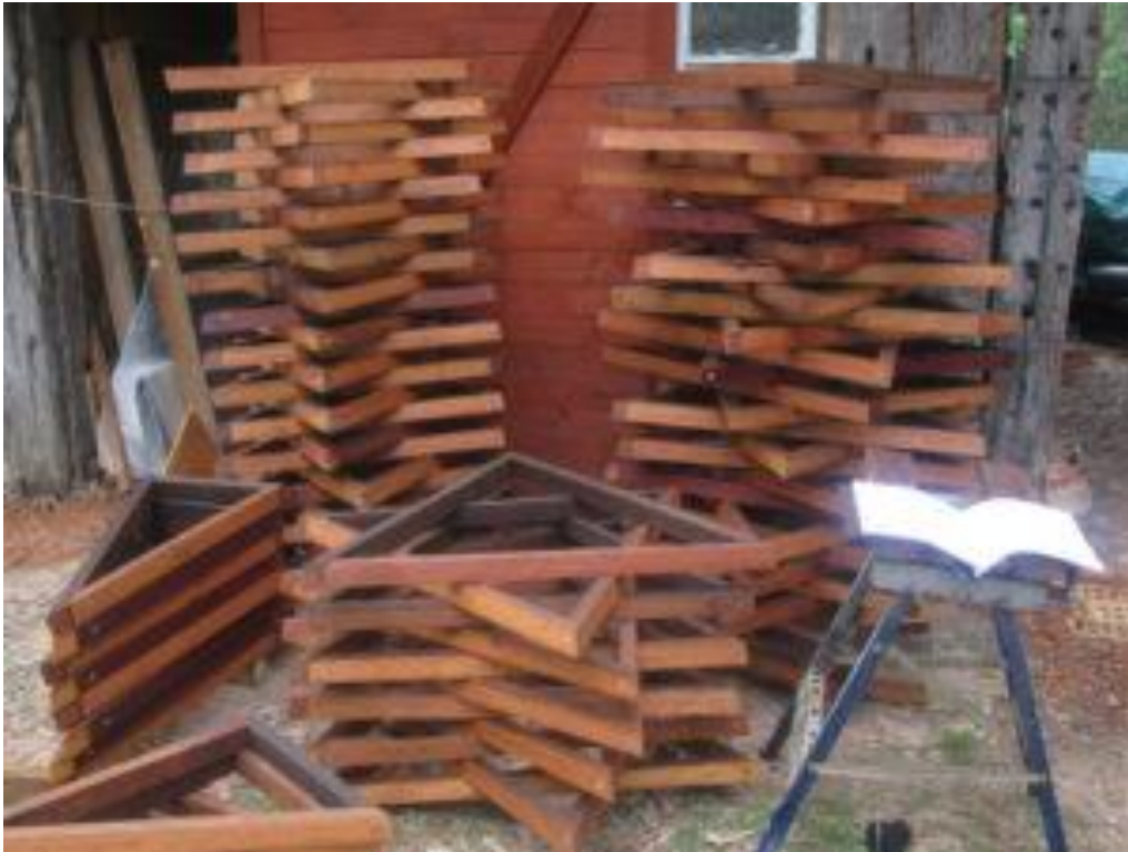
Anthony has started to build a rounded dome built out of triangles of wood in our car-park in April 2017. He calls it a Geodesic Dome.
