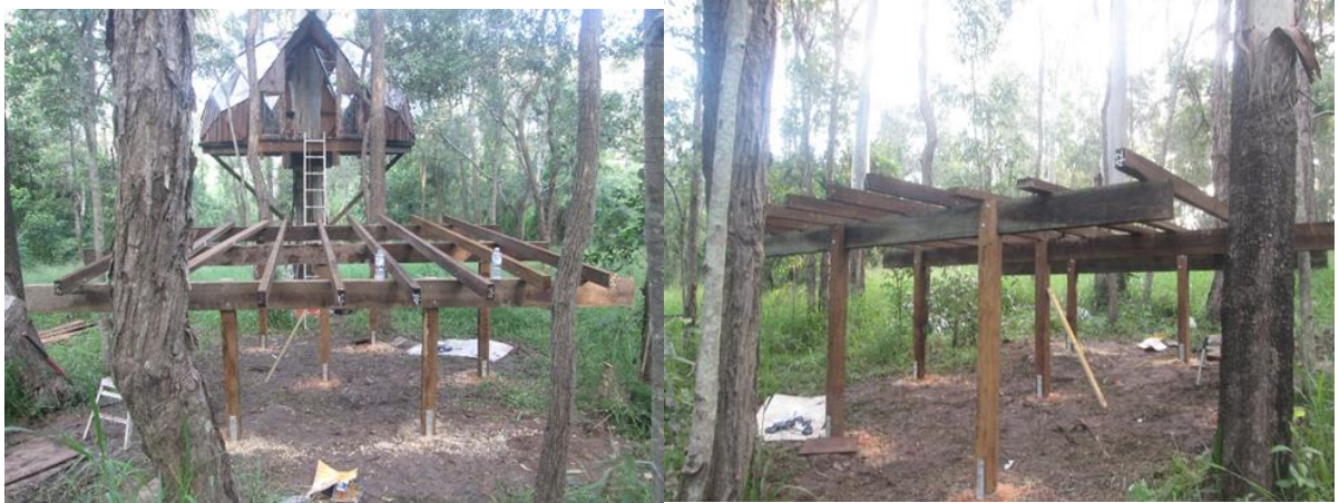
The twelve vertical posts along with the bearers and the rafters for the deck.
