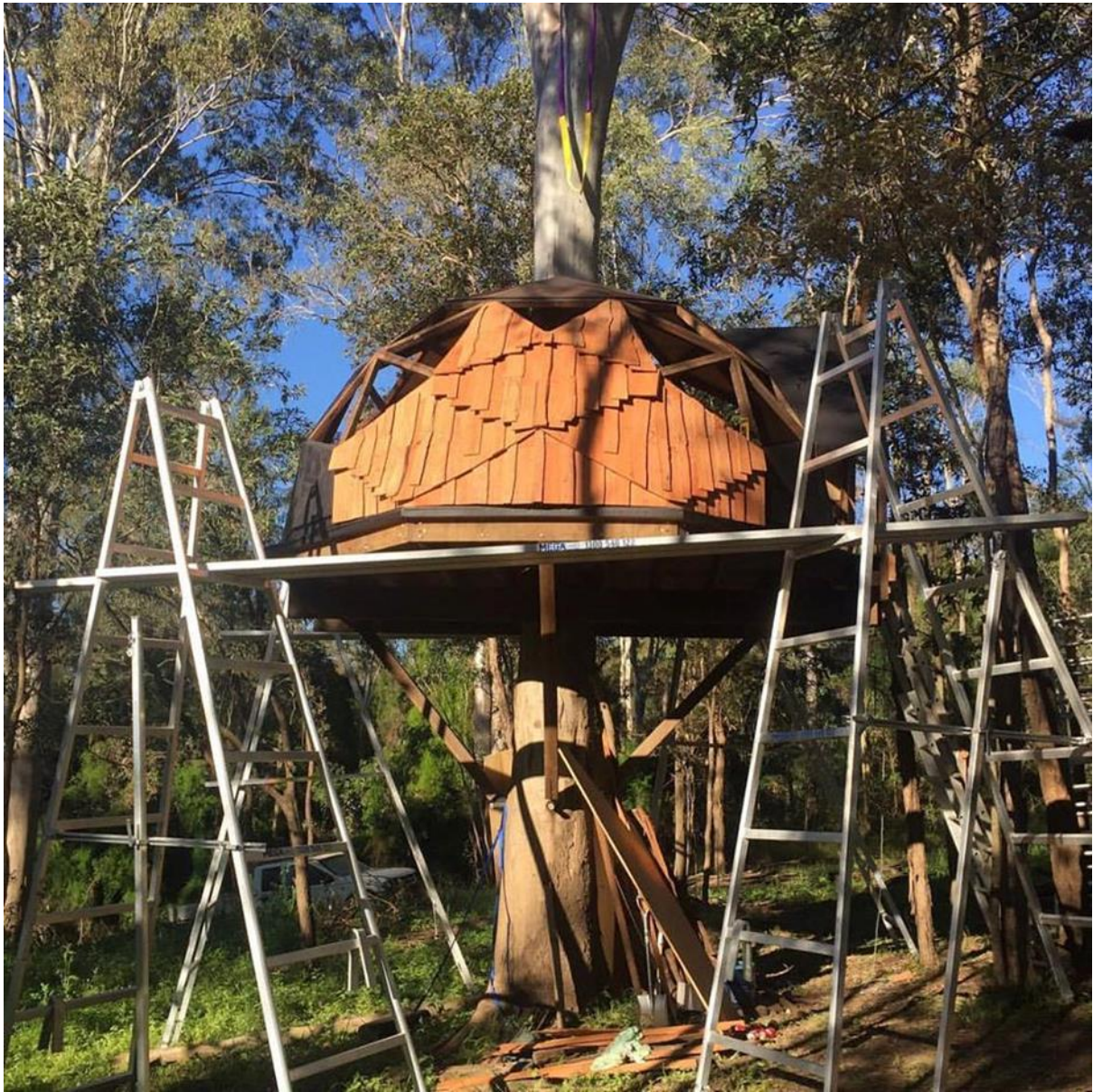
Shingles going on the Geodesic Dome
