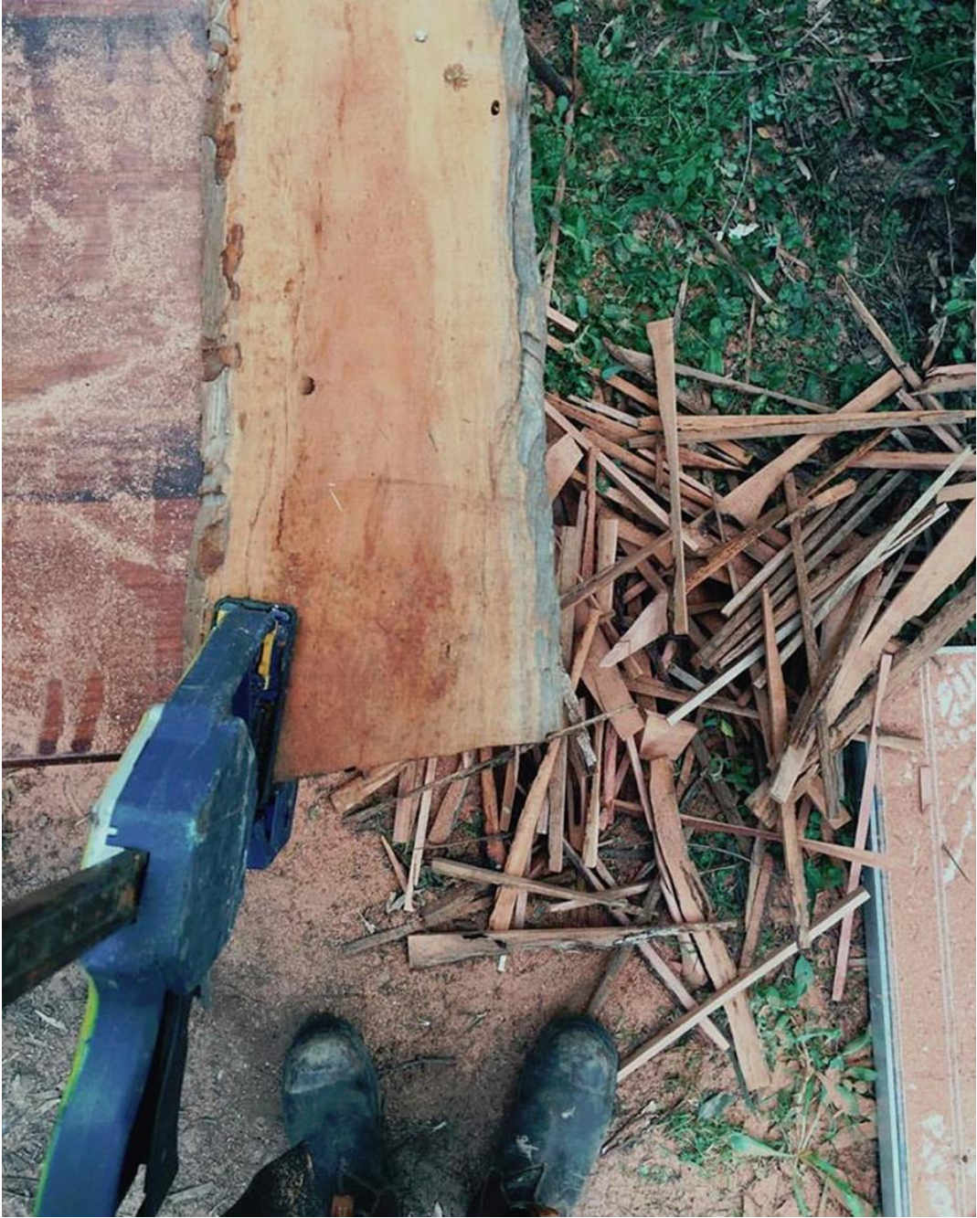
Trimming the live edge of the shingles
